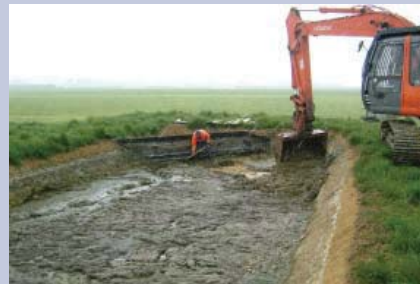
Excavator loading the dried sludge
