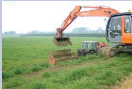
Excavator loading a muck spreader
